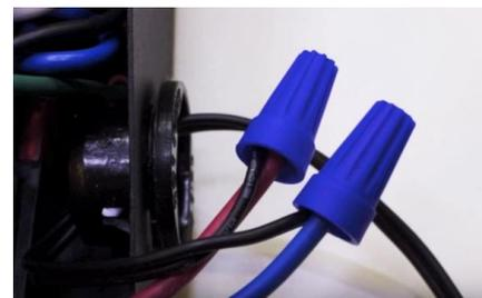
**5** Connect transformer to low voltage LED wiring using wire nuts: red (+) positive, blue negative (-)
