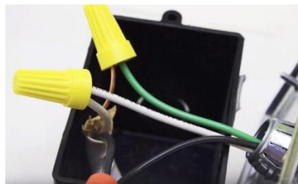
**4** Connect in-wall cables from switch to transformer using wire nuts: black (+) to 120V, green to ground, and white (-) to neutral
