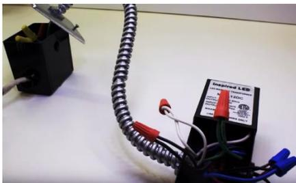
**3** Using in-wall rated or armored cable, run wires from compatible wall switch through wall box or directly to location of transformer
